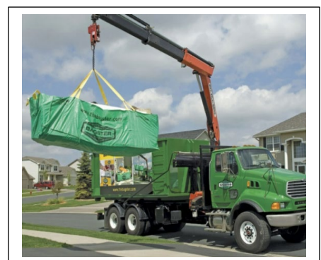
Do not place dumpsters, flexible or solid on any part of a sidewalk
